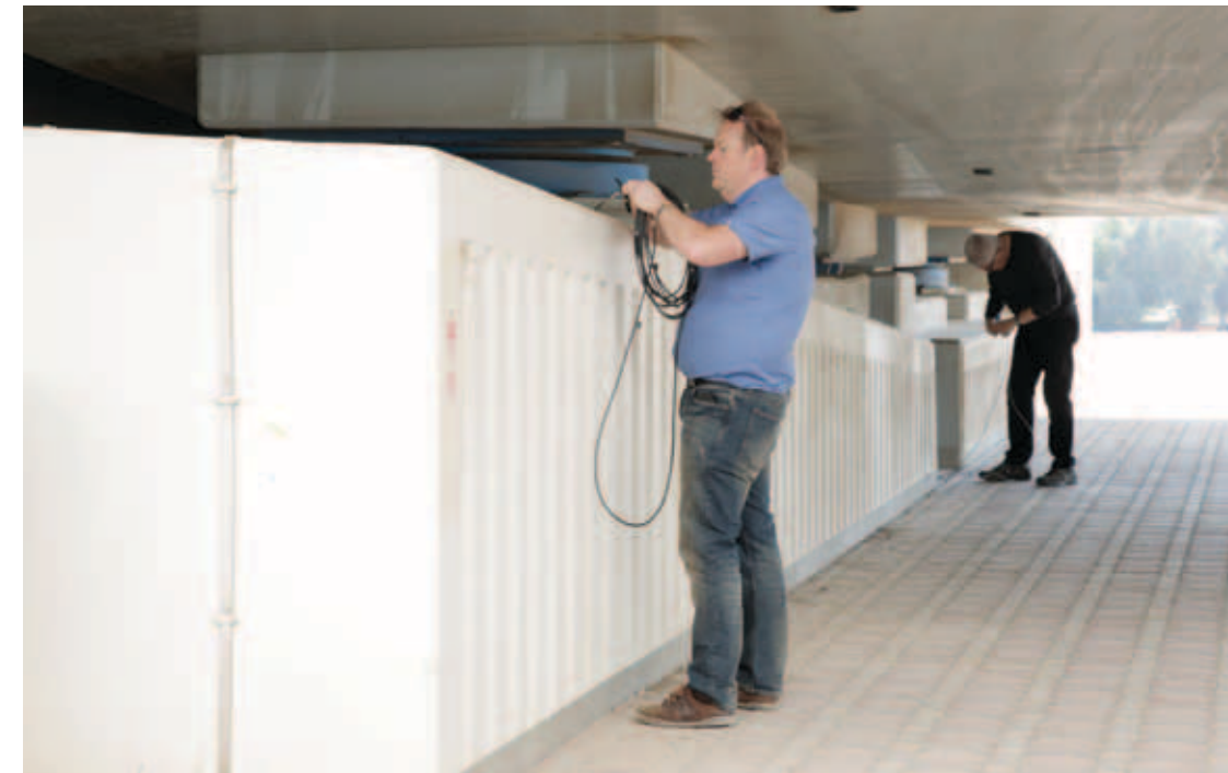
January, 2014. Sound engineer Scott George and Bill Fontana place accelerometers and other sensors throughout the bridge structure.
